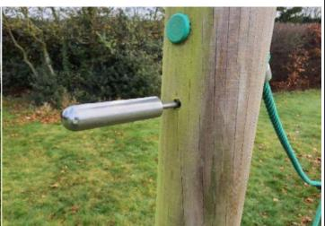
**Finding:** There is/are finger entrapment/s in the post due to **Action:** Provide missing components to remove entrapment missing components and the item fails to meet the requirements of BS EN 1176 Part 1 4.2.7.6 Entrapment of fingers
