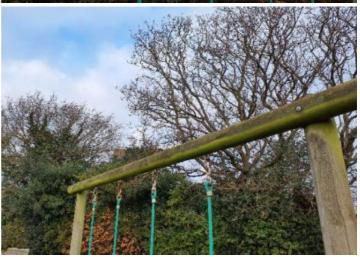
**Finding:** The inspector has some concerns about the internal condition of the timber crossbeams and was unable to verify the structural integrity without further testing. We recommend a Resi-PD survey to establish the condition of the timber at it's core. **Action:** Contact th further information
