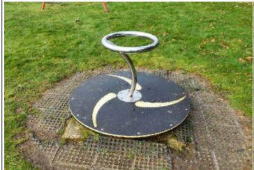
**Finding:** The raised concrete base forms a hard object within the falling space of the equipment and there is also insufficient surfacing provided in contravention of BS EN 1176 Part 1
