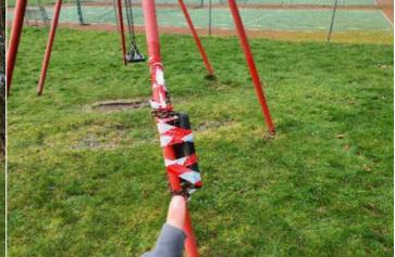
**Finding:** There is minor distortion damage to one of the legs **Action:** Monitor for any further deterioration and repair or replace as required
