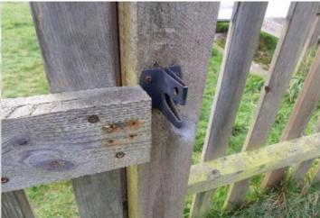
Finding: The gate latch is damaged or missing Action: Repair or replace
