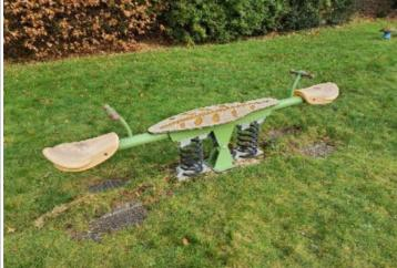
**Finding:** The concrete base/ timber edge forms a hard object within the impact area of the equipment in contravention of the requirements of BS EN 1176 Part 1
