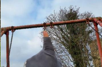
Finding: The connecting pin is showing signs of wear
