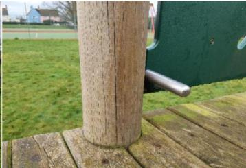
Finding: There is/are finger entrapment/s in the barrier and Action: Monitor - No remedial work recommended the item fails to meet the requirements of BS EN 1176 Part 1
