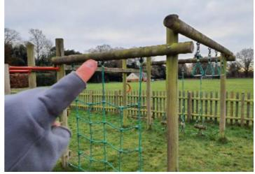
**Finding:** The inspector has some concerns about the internal condition of the timber crossbeams and was unable to verify the structural integrity without further testing. We recommend a Resi-PD survey to establish the condition of the timber at it's core. **Action:** Contact the further information
