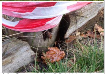
**Finding:** The timber on this item has severe rot and there are protruding bolts present
