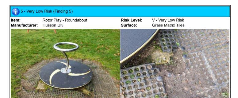
**Finding:** Fixing Pins have been installed in the impact areas **Action:** Remove pins from impact areas of the grass mats
